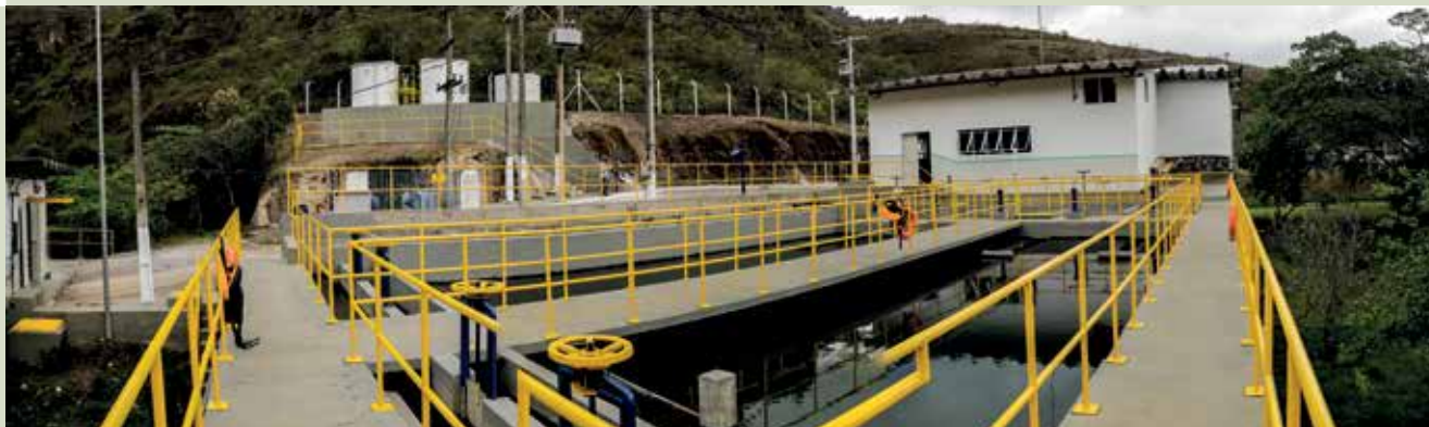
Itacolomi Water Treatment Plant (WTP). Saneouro – Ouro Preto/MG
